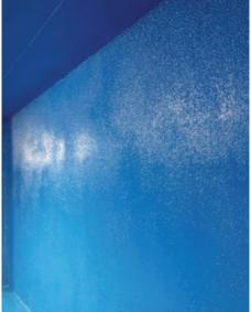
Our versatile coating PROGUARD CN 200 is easily applied by airless spray. Due to its high sagging limit, PROGUARD CN 200 can also be sprayed on vertical surfaces with a layer thickness of 1000 µm - this allows applications in just one coat and one pass, even for complex surfaces. The coating cures completely within a few days; the tank can be filled and put into operation rapidly.
