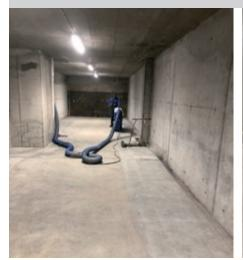
The concrete surfaces are prepared using a dustfree technology. Blowholes and fixing holes are covered with a high-quality filler.
