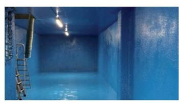
Concrete fire water and sprinkler tanks for large buildings require reliable protection against leaks. Uncoated concrete becomes porous due to the massive exposure to water. In order to prevent the concrete from damage and to provide long-lasting protection, indoor concrete tanks should be coated with a suitable protection system.
