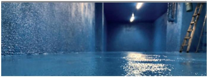
Large residential buildings or factories need sufficient storage of fire extinguishing water in case of emergency. Our partner "Strohbeck GmbH" protects the indoor concrete tanks with our coatings – providing a durable, effective protection against the large volumes of water.
