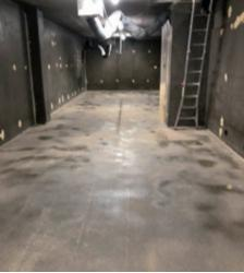
Firstly, the concrete substrate is primed with our base coat CP-SYNTHOFLOOR 8010. Quartz sand is sprinkled onto the wet layer, which forms an anchoring profile for the following layer. Floor unevennesses are levelled by an additional scratch coat (primer enriched with quartz sand).
