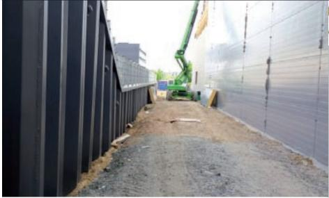
The polyurethane topcoat PROGUARD 169 provides long-term weather-resistance and UV-stability. The customer chose the special color DB 703 MIO (micaceous iron ore). Our 1-layer system was applied with a dry thickness of ca. 90  $\mu$ m.
