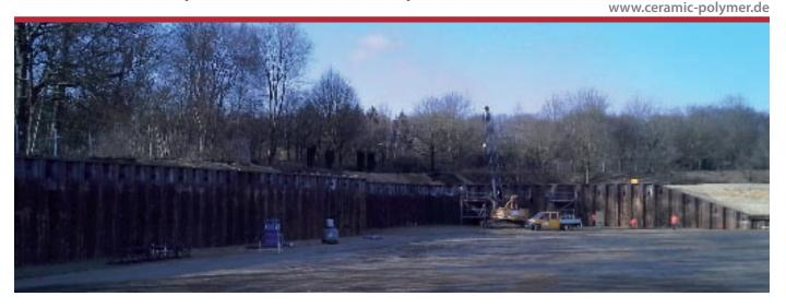
Hamburg/Germany: A wholesale trader for frozen foods and canteen kitchen technics has built an extensive sheet pile construction as surrounding of its new warehouse, which is under process. The company "Strahl- & Sanierungstechnik GmbH & Co. KG", located in Wildenhorst/Germany, coated the sheet piles with our products for the reliable protection against corrosion and weathering.
