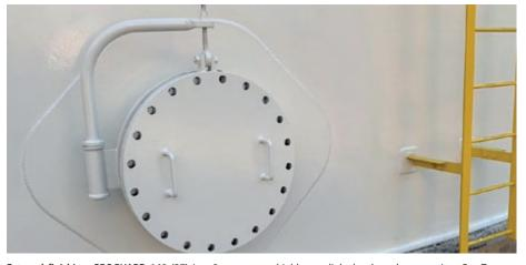
**External finishing: PROGUARD 169 (37)** is a 2-component highly-crosslinked polyurethane coating. Our Topcoat provides resistances according to ISO 12944-2, corrosivity class C5. Therefore, it is the ideal product for demanding industrial environments. **PROGUARD 169 (37)** is available in RAL and NCS colors, it can be applied in one thin layer and shows fast curing. In this case a layer of 70 μm was applied by airless spraying.
