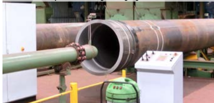
► Internal coating of cooling water intake risers for extensive FLNG-Project in Australia – only available in English language
