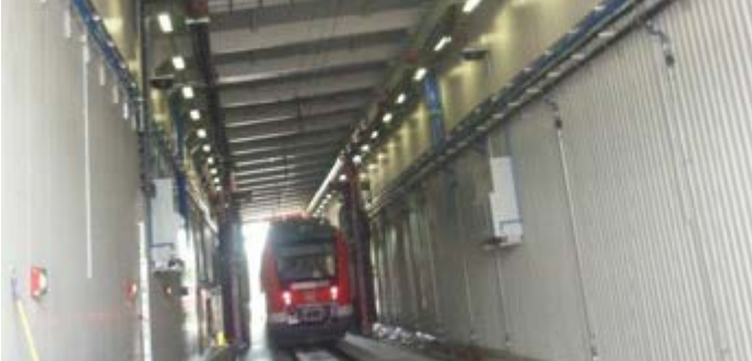
► Coating of a wash tunnel of "German Railways" – resistant against acidic detergent
