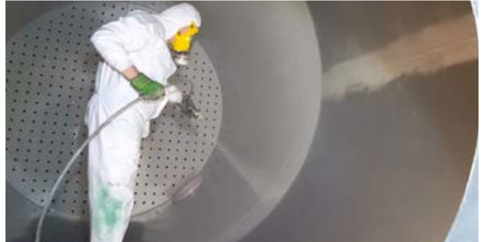
► Internal coating of gravil filters and activated carbon filter tanks
