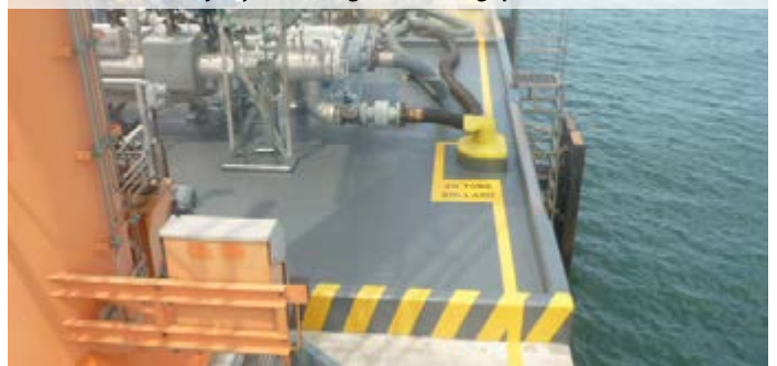
► Skid-proof and A-1 chemical resistant - PROGUARD CN-1M for a maritime oil jetty on Jurong Island / Singapore
