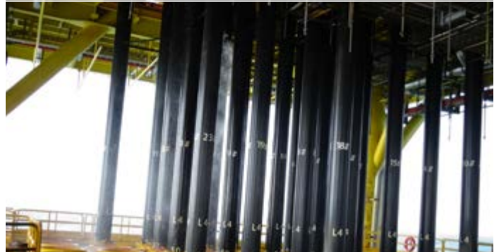
► External coating of risers and injection pipes for oil platforms in China
