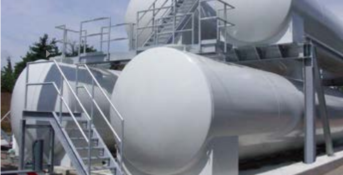
► Internal coating of storage tanks for methanol
