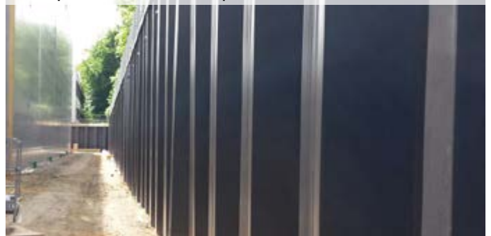
► Durable corrosion protection and weathering resistance for extensive sheet pile construction (1.800 sqm)
