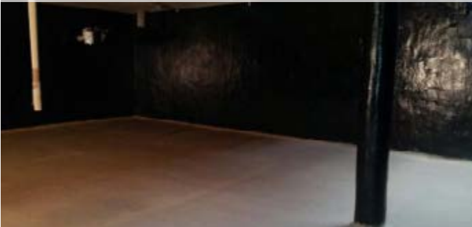
► Coating of storage room for aggressive bio-waste with Proguard CN-1M! - only available in English language
