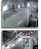
The heavy damaged and corroded surface was prepared adequately by grit blasting. Susceptible and defective spots were refinished with our special repair grout **Proguard GS**.
