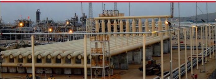
During the extraction process, natural gas is very humid and therefore highly corrosive. Due to the high pressure and absorbed stones, extreme abrasion occurs on the internal walls of the whole pipeline system.
