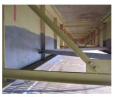
Our coating product Proguard 96 (color "sand yellow") was applied by airless spraying on the prepared substrate. One layer of 200  $\mu m$  is adequate to provide an outstanding corrosion protection.
