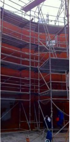
Both open steel tanks had wall and floor surfaces of 1.000 m<sup>2</sup>. After pre-treatment (sandblasting, SA 2 ½) the coating was applied simply by airless spraying methods.
