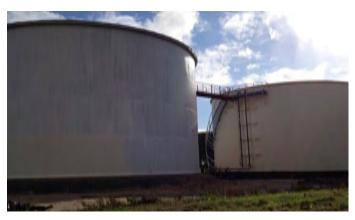
Until further processing, the highly corrosive liquid is intermediately stored in these tanks with a temperature of 60°C. Therefore, high requirements for corrosion protection are placed in this field of application.
