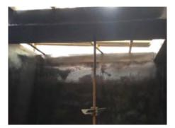
The concrete walls and ceilings were coated directly with our product Proguard CN-1M. No previous use of a primer is necessary when the application is conducted by airless spraying methods.
