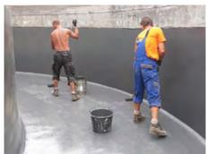
ISDW GmbH started the following works on the inner basin. To achieve a smooth surface the wall area was firstly treated with "CP-Synthofloor Beta 8016" as scratch coat. After the curing the coated walls were milled to prepare the substrate adequately for the application of the primer. For the best protection the edges were sealed additionally.
