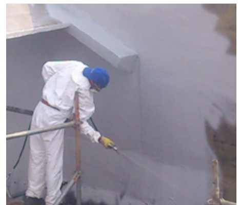
Application of the coating PROGUARD CN 200
