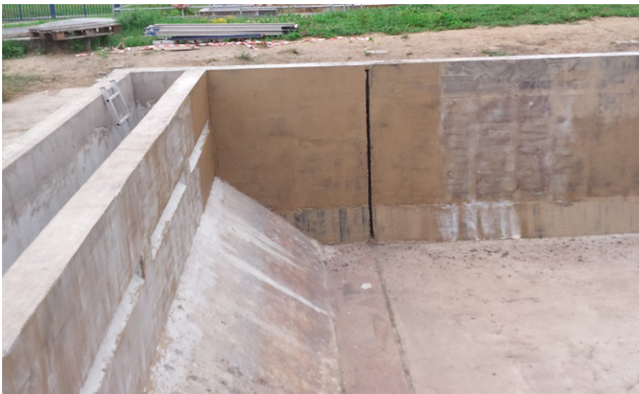
Rebuilt top edge, application of the primer
