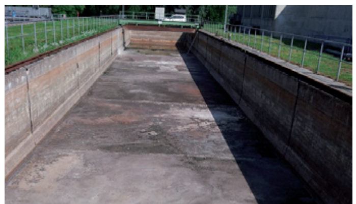
Buffer tank before refurbishment
