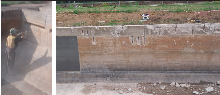
Grit blasted area, loose concrete was removed
