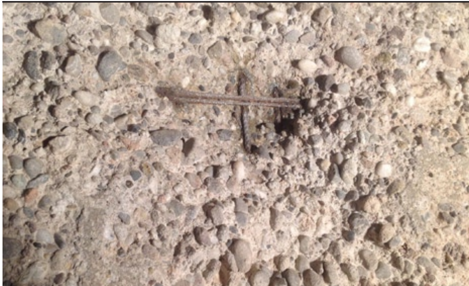
"Washed-out-concrete-effect" - caused by aggressive acids in the ensilage
