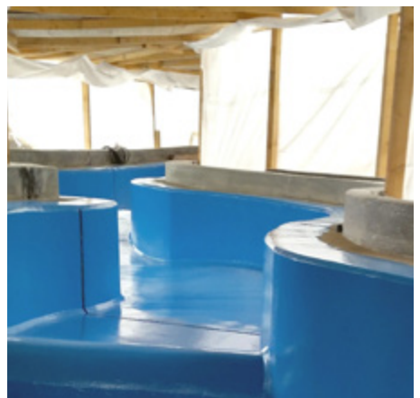
After curing of the prime coat the surface was grinded and the coating product PROGUARD CN 200 was applied
