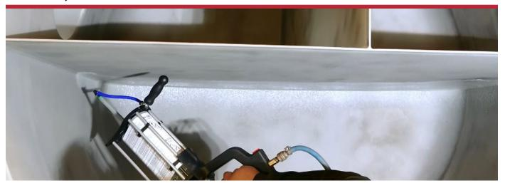
The company "Zacosin<sup>®</sup> the surface experts", located in Gladbeck/Germany, uses for comprehensive corrosion protection of small special tanks our premium coatings with cartridge application system. This application method facilitates a clean and cost saving coating for small projects and hardly accessible areas. The cartridges are resealable; the remaining material can be utilized for at least 6 months.
