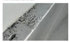
The cleaned areas which are heavily damaged by corrosion were filled and smoothed with our special composite putty PROGUARD CN 200 THIX. This filler material is applied by rake or brush. It forms the optimum sealing of sensitive zones such as edges, corners and welding seams.
