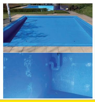
Coatings, which are being applied in pools and tanks for chlorinated water, have to provide different resistance properties. For constant operation the waterproof sealing to the concrete substrate is equally important as a reliable stability against chlorine. For pools a good resistance to UV radiation is furthermore requested.
